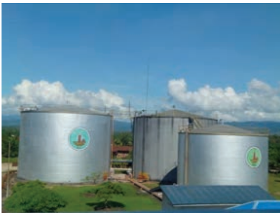
CPO tanks in PT NJL
