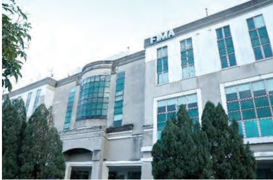
Plaza Damansara Building
