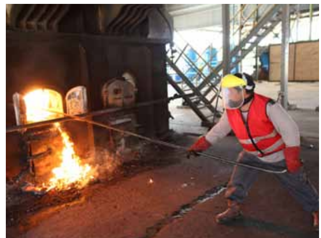
Boiler handler at PTNJL
